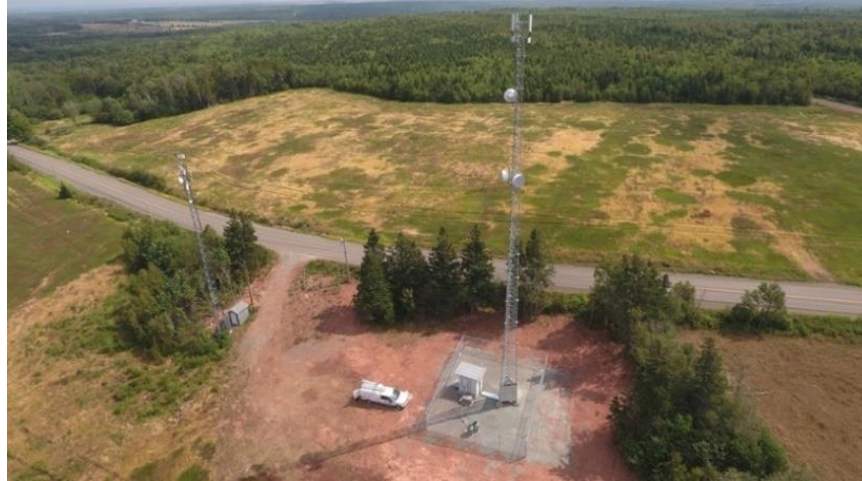
Figure E – Proposed Xplornet 45m Self-Support Telecommunications Tower
