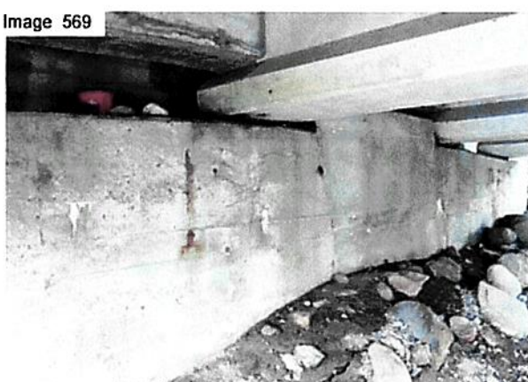
Diaphragm and girder north end damage
