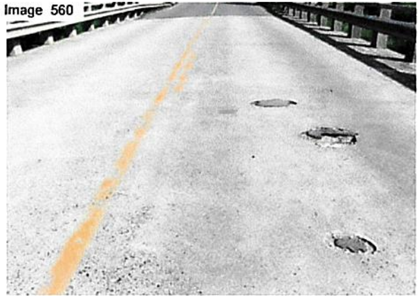
Asphalt on deck typ.
