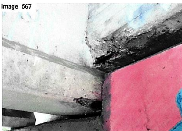
Diaphragm and girder north end damage
