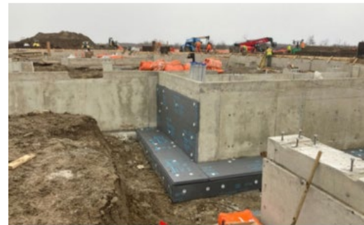
Insulation work around footings
