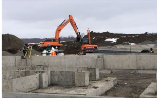
Foundation Works stripped in North / West wing
