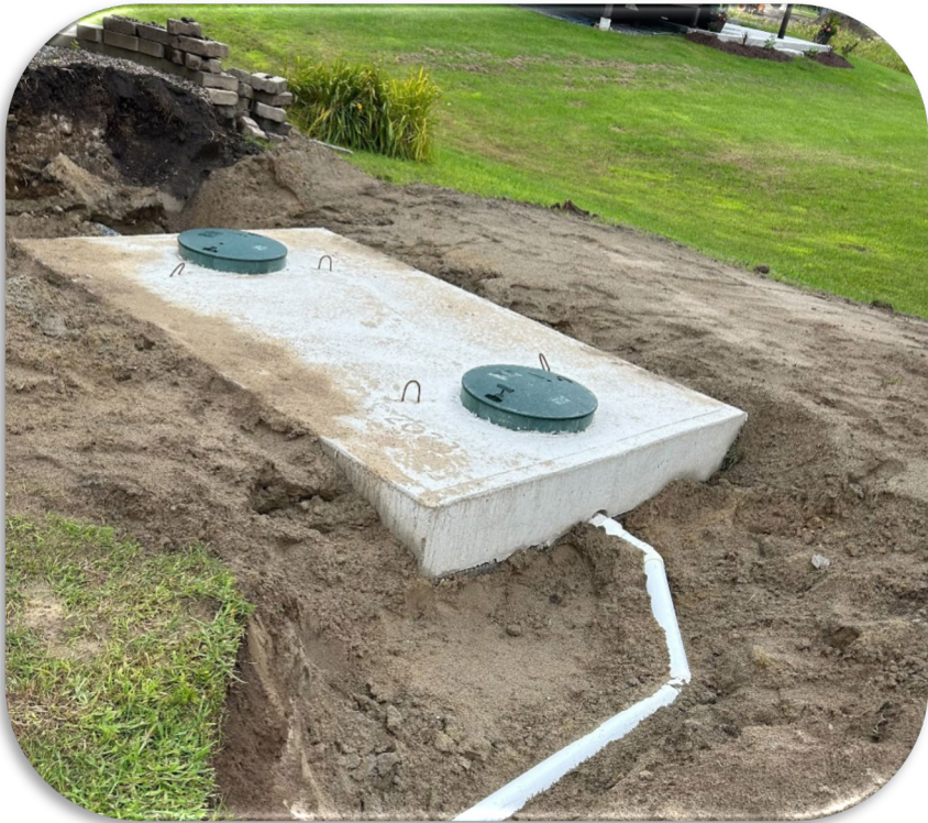
Tank replacement with Elmer Construction Township of Edwardsburg/Cardinal
