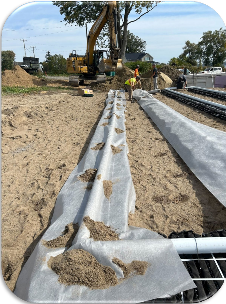
Installation with Easton Excavation Township of Front of Yonge
