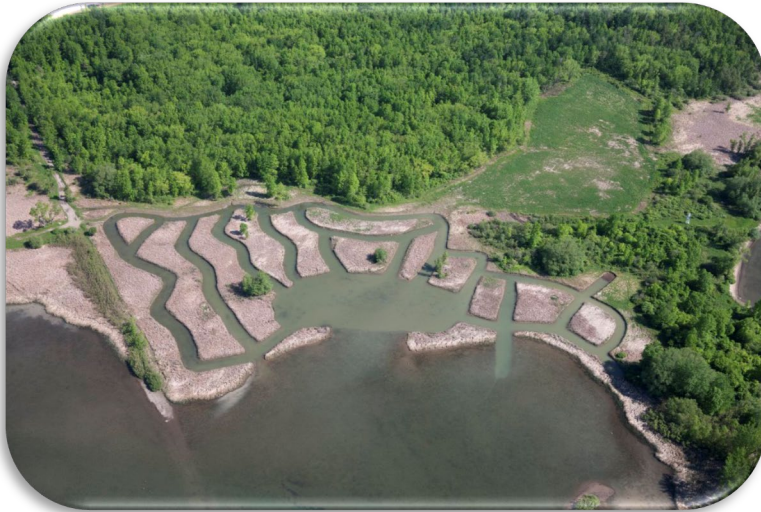
Fish Habitat Compensation Project, Port of Johnstown
