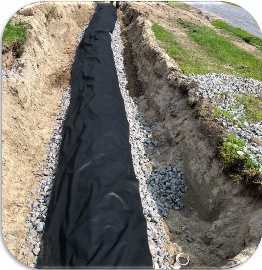
Installation with Ken Beck Excavation Township of Augusta
