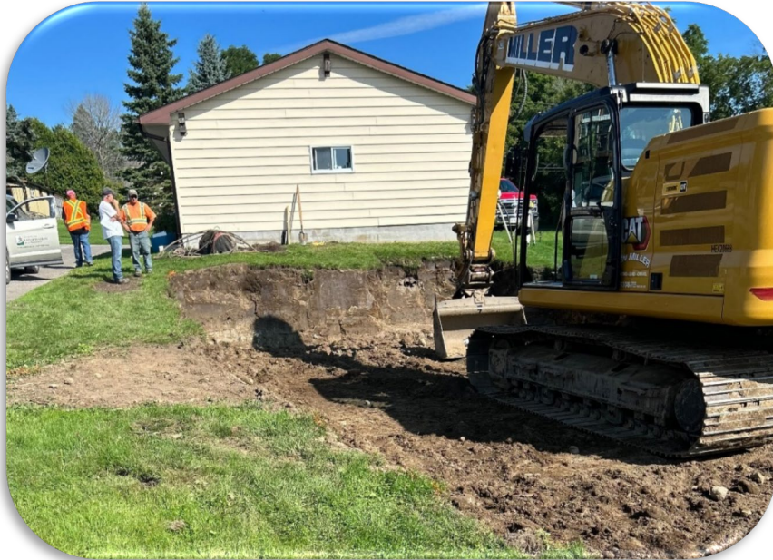
Excavation Inspection with Miller Excavation Township of Elizabethtown-Kitley
