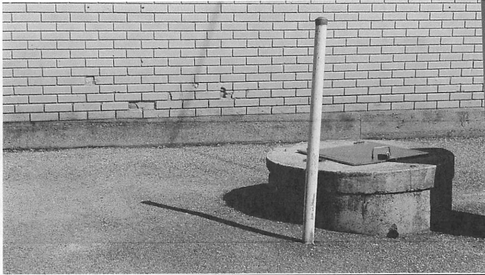
2022-A5 – Damaged Brick on Front Elevation
